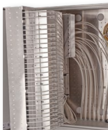
Cable/duct management view
