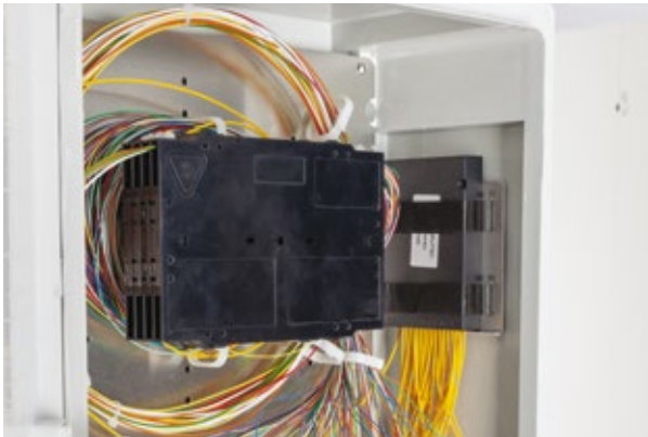
PLC splitter placement
